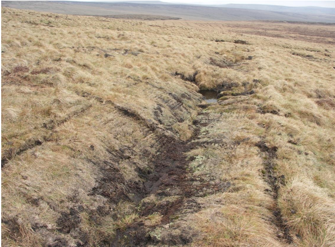
Figure 1.7a: Photo of reprofiled grip.
