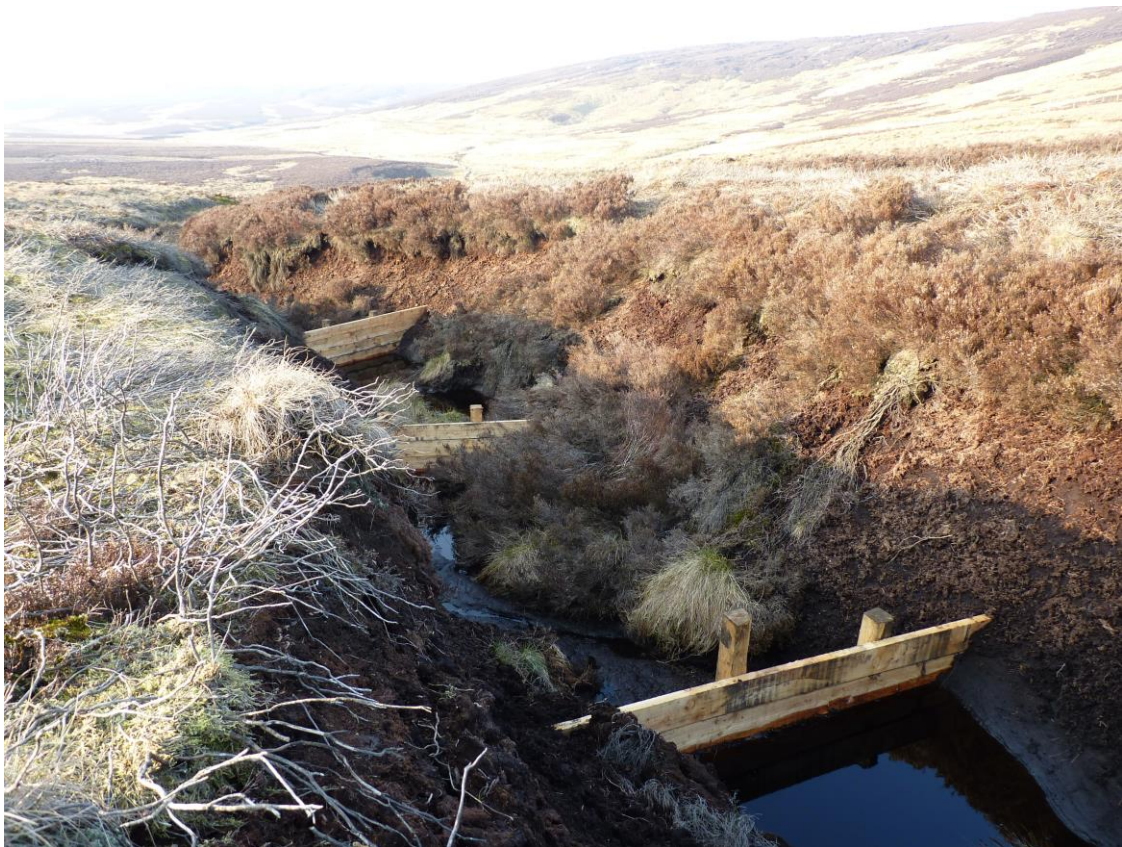
Figure 1.8 Timber sediment trap
