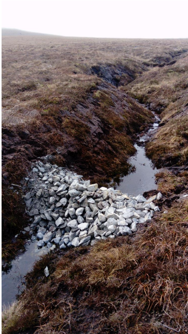
Figure 1.10 Photograph of Stone sediment trap
