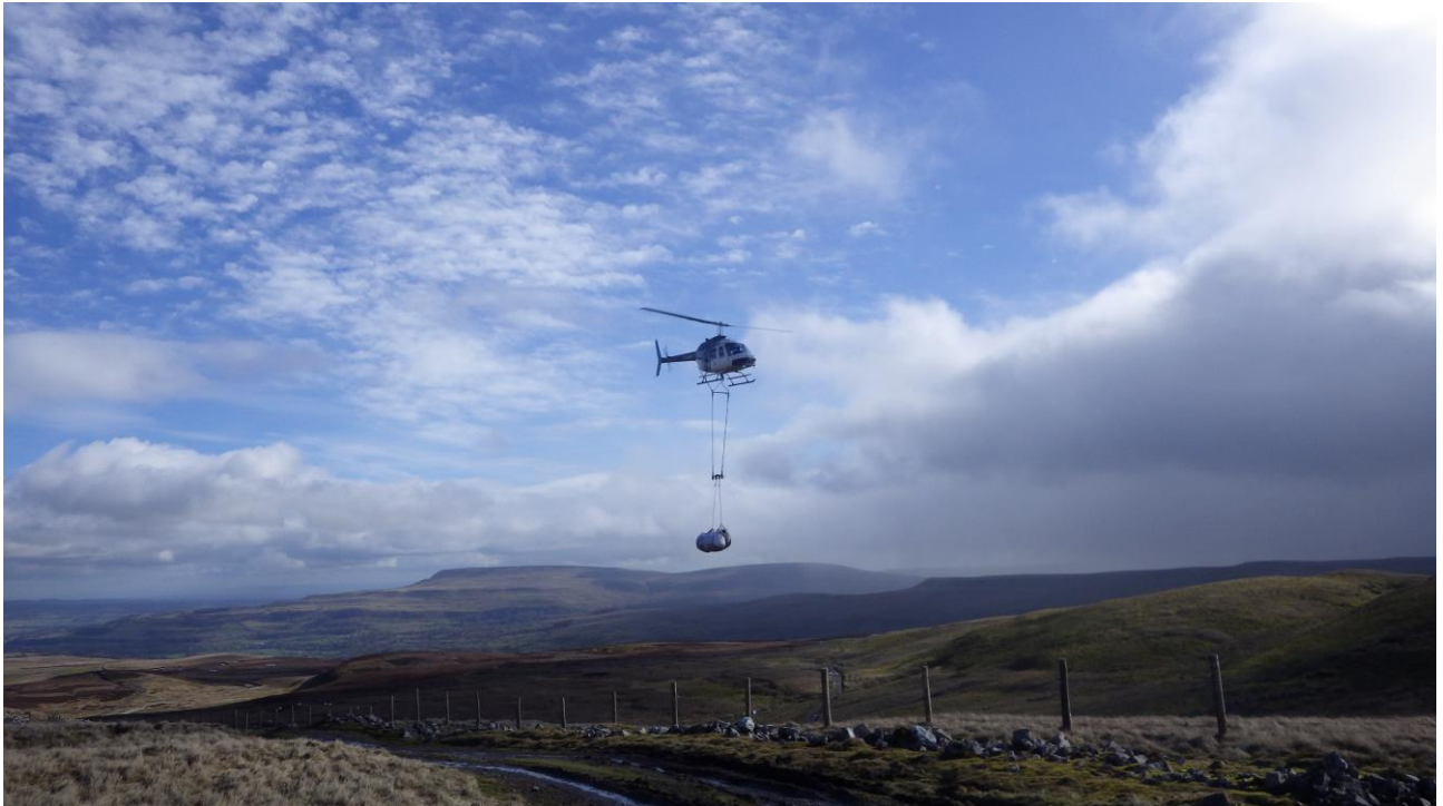
Figure 2.6 Photo of brash dumpy bag being lifted by helicopter
