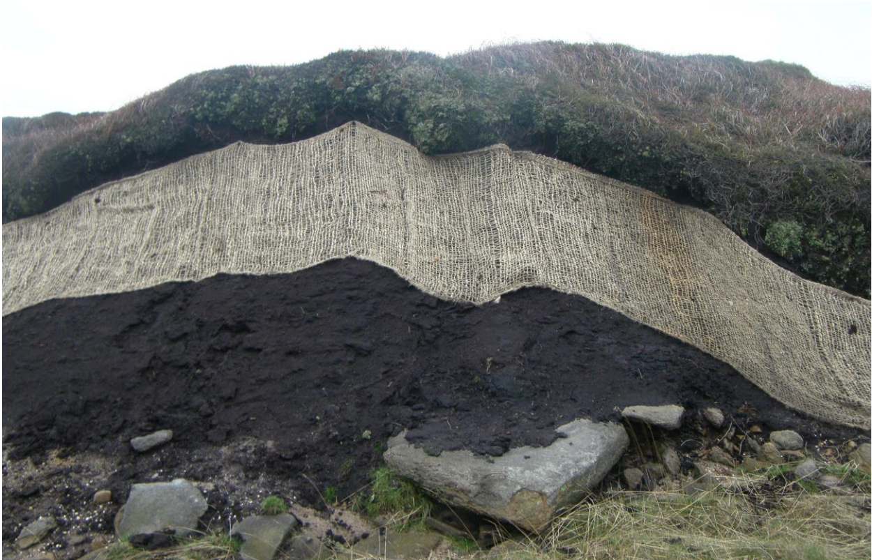
Figure 2.4 photo of a geo-textile treated slope
