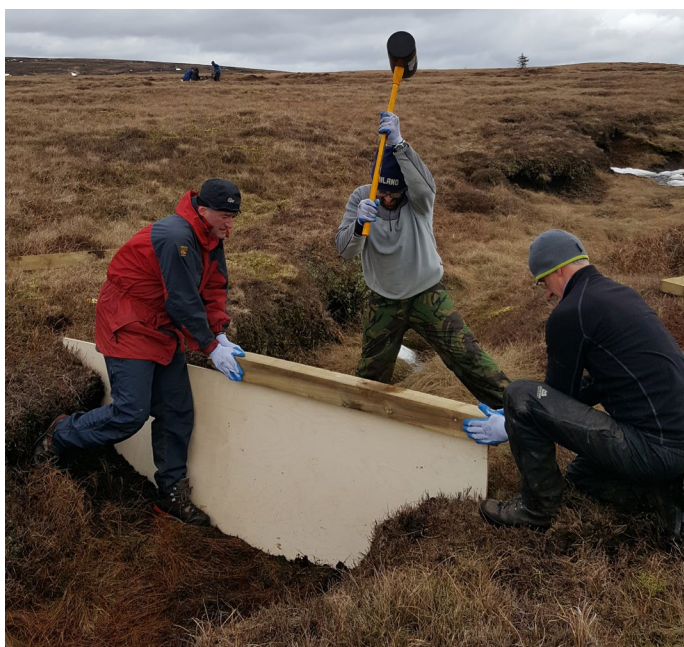
Figure 82 Hammering in a ply sheet dam. Note, the C-bar and use of rubber maul. © Emma Shuttleworth
