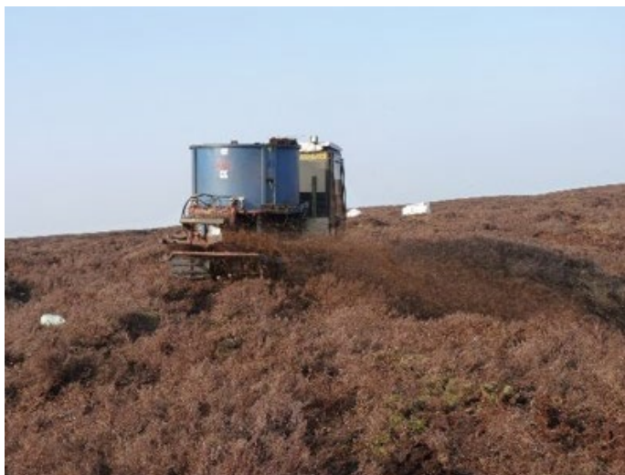
Figure 135 Brash being applied to the sides of eroding gullies by specially adapted low ground pressure machinery © Yorkshire Peat Partnership
