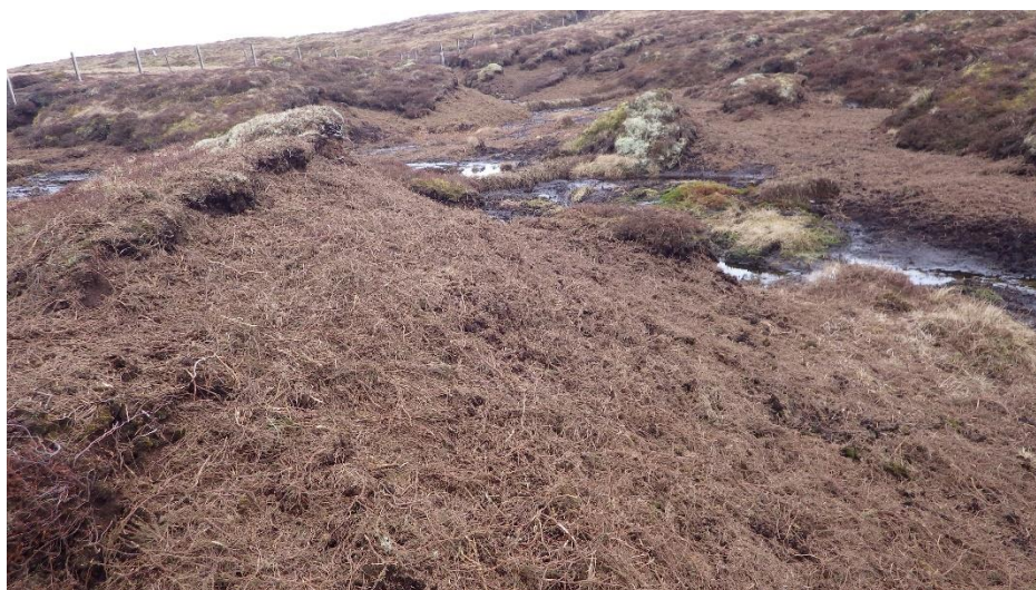
Figure 11: Brushed, re-profiled slope
