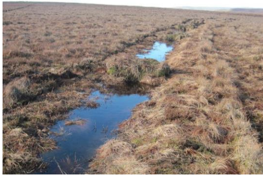
Figure 6: Blocking grips and gullies with peat dams
